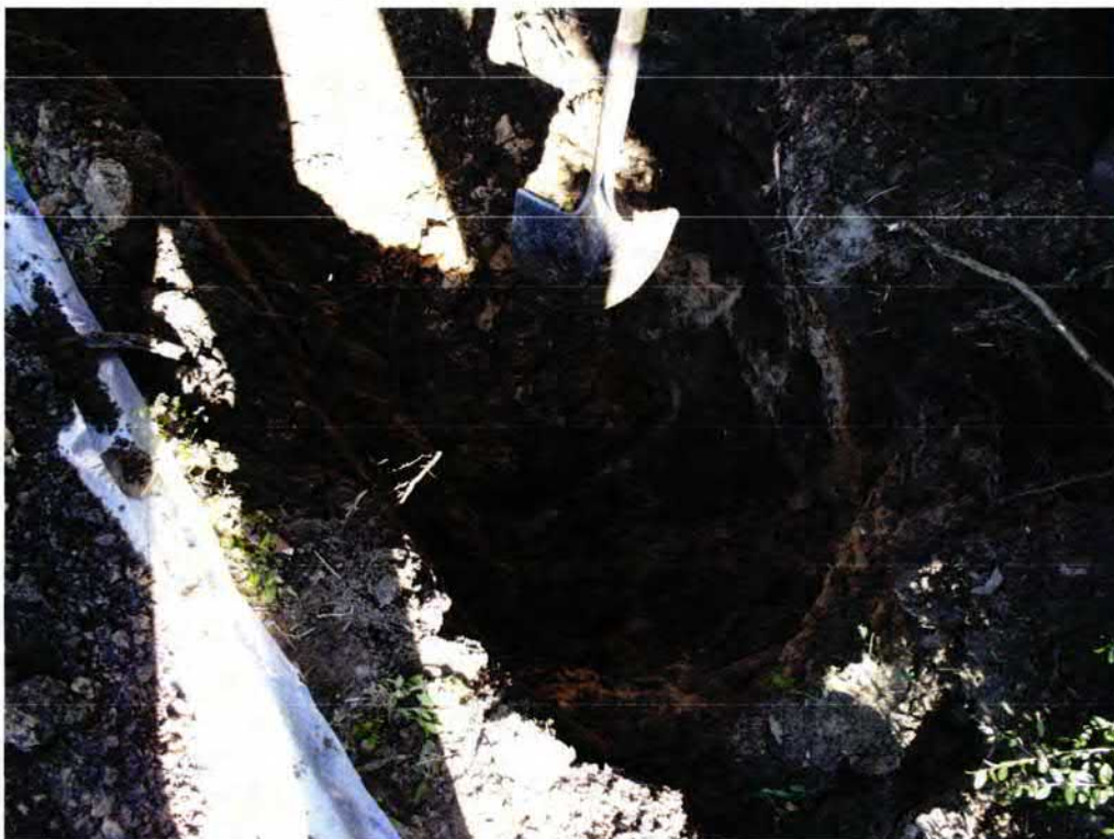
Picture 2: UST 425Elderberry excavation in progress.
